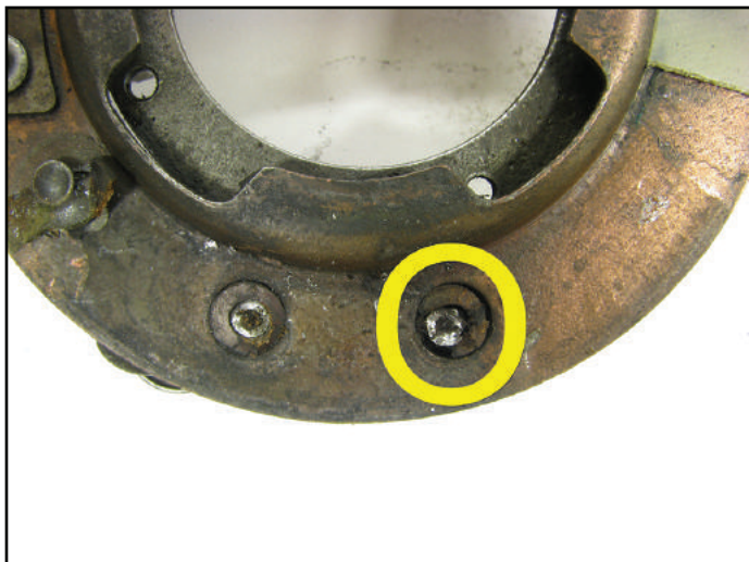
Figure 5 – After removing the positive brush's holder, you can see the burned rivet insulator.
