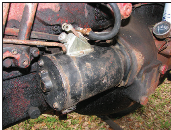
Figure 2 – The actuating lever linking the mechanical switch to the starter's actuating rod was missing.
