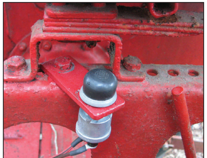
Figure 7 – A push button starter switch was installed just below the driver's seat on the left side.
