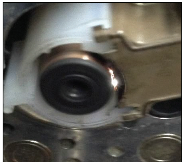
Figure 7 – Under the same load and RPM but with the belt slipping, the arcing is obvious.
