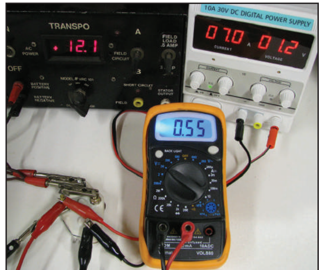
Figure 5 – The regulator tester activates the 22-SI regulator's power transistor. The power supply passes 7 amps of current across the transistor's junction. The DVM measures Vsat.
