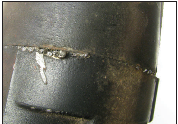
Figure 4 – The bits of molten metal on this 28MT intermediate housing got my attention when I checked it. I suspected contact resistance as being the cause.
