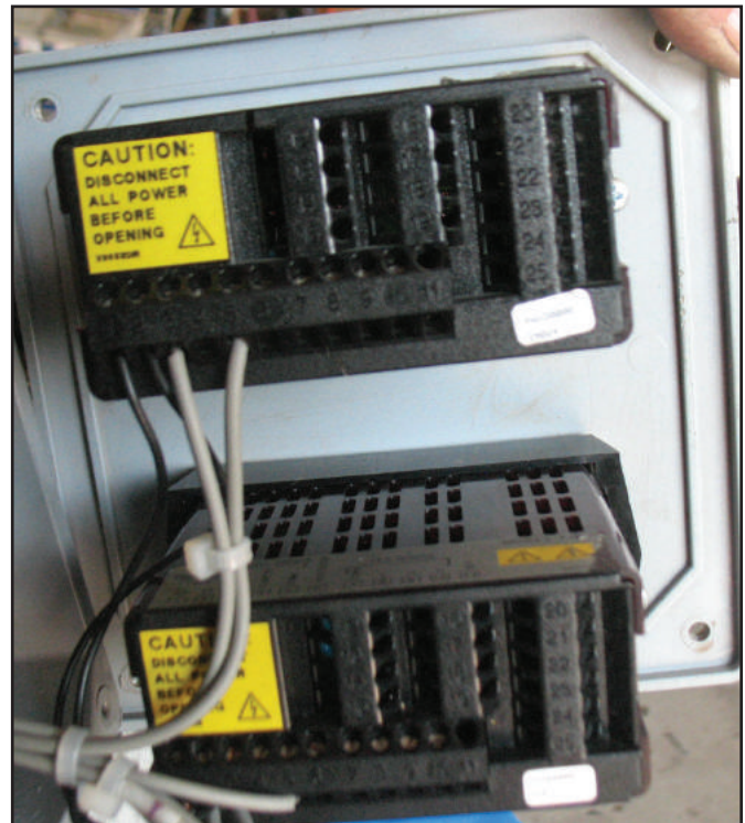
Figure 3 – This rear view of the digital meters gives you some idea of how many different inputs this meter is capable of processing.
