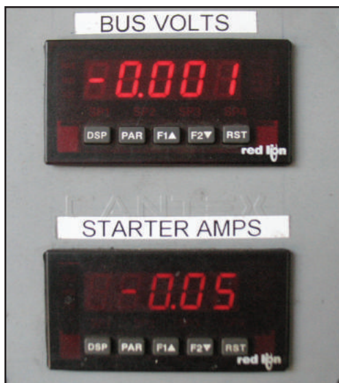
Figure 2 – In this close up of the digital display, you can see programming buttons on the bottom of each meter.
